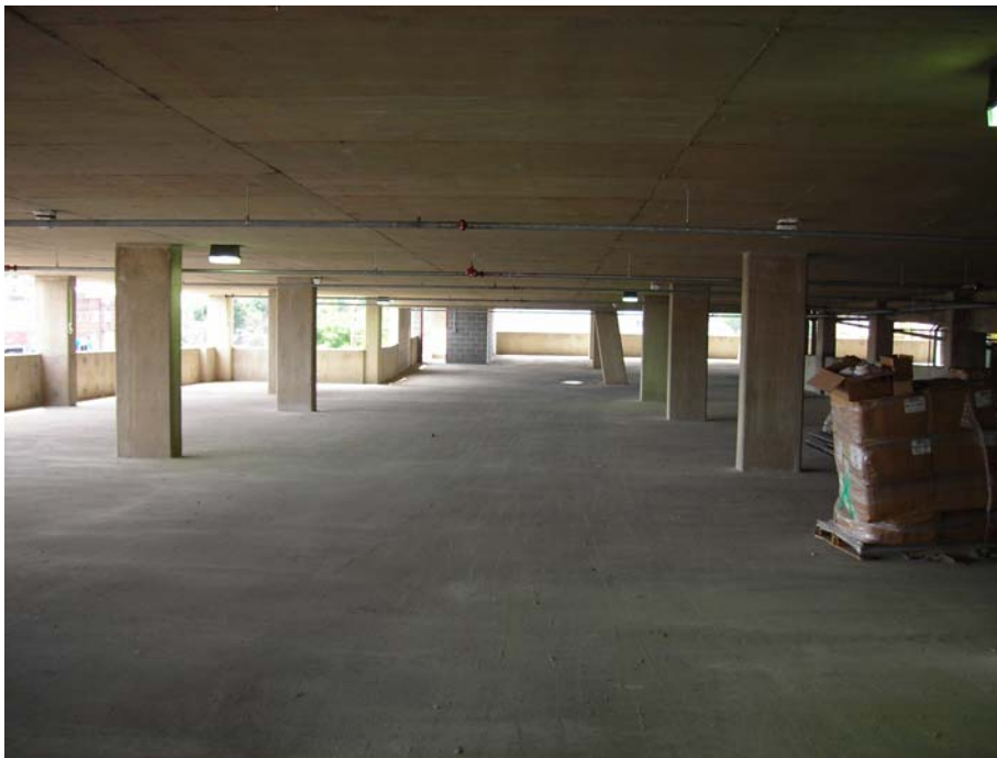
Photo 6: Interior View of the parking garage.
