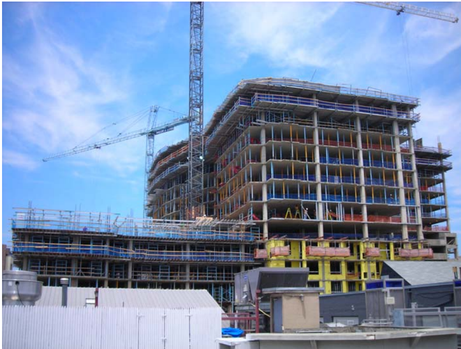
Photo 1: Overall view of Southeast elevation of Silver Spring Gateway.
